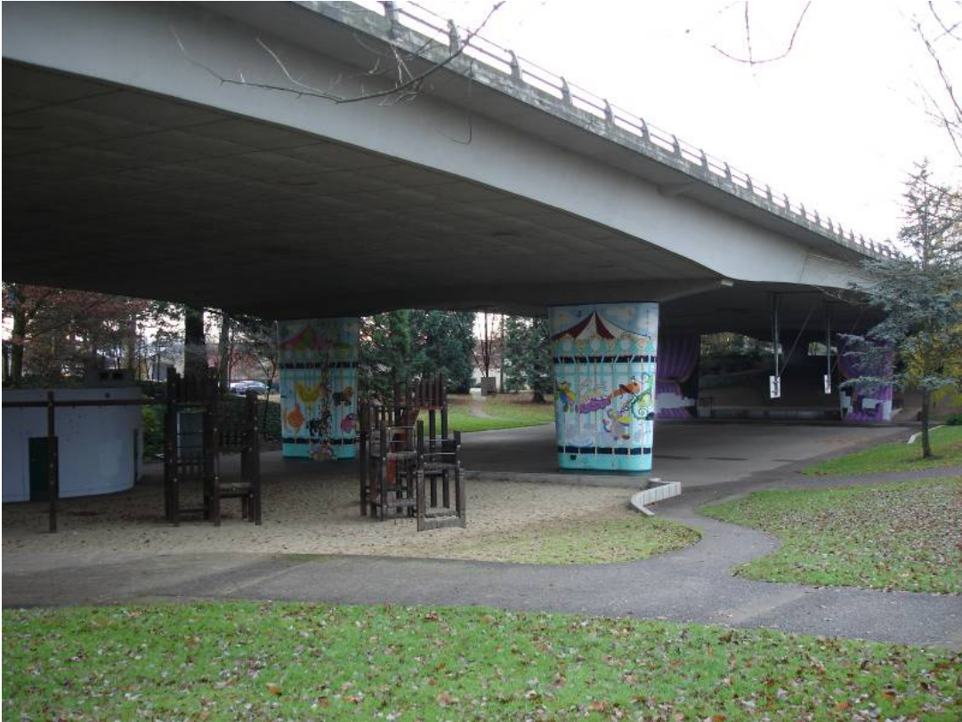
Existing Restroom and Playground Facing Southeast
